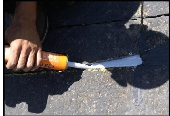
**3)** Seal over the yoke to fill the groove.
