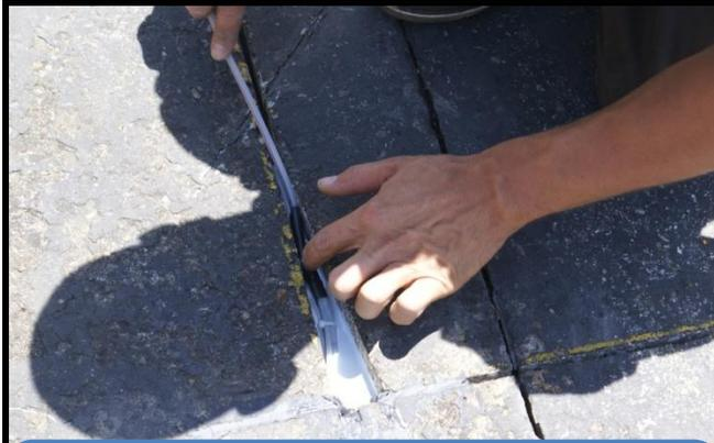
**2)** Gently press the yoke into the bead of sealant, the yoke should be resting on a small layer of sealant.
